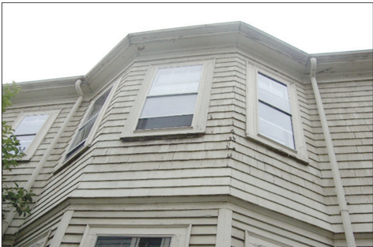
Old wood gutter, soffit and fascia that needed replacement.
