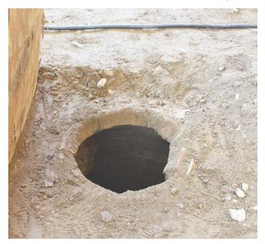
During the excavations at the rear if the basement of the West Branch Library a circular well, which had been covered and unused for decades has been discovered. It seems to be in good condition but with town water supply a well was no longer needed.
