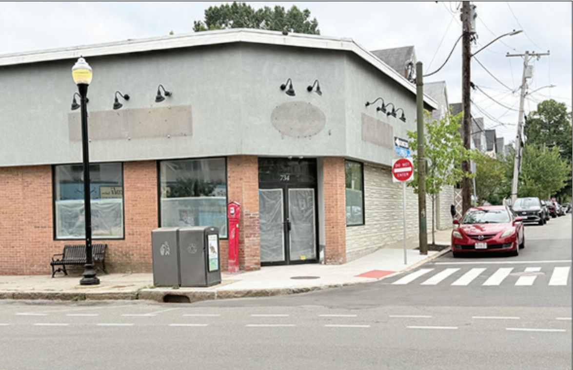
The new location at 285 Boston Ave., Medford, a former convenience store.
