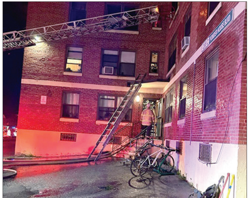
An aerial ladder and a ground ladder are seen raised to the second and third floors of 268 Powderhouse Blvd.
