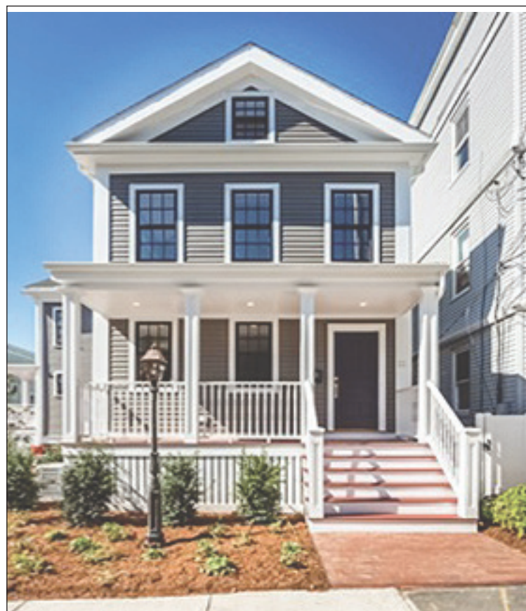
The freshly renovated award winning house at 22 Linden Ave.
