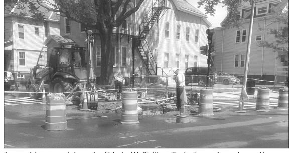
A water main burst open at the intersection of School and Medford Streets Tuesday afternoon. Apparently, an outside construction crew hit the water main and water gushed out all over the area, causing a small flood. It appeared that an outdoor contractor hit the water main accidentally while digging in the area, breaking open the water main.
