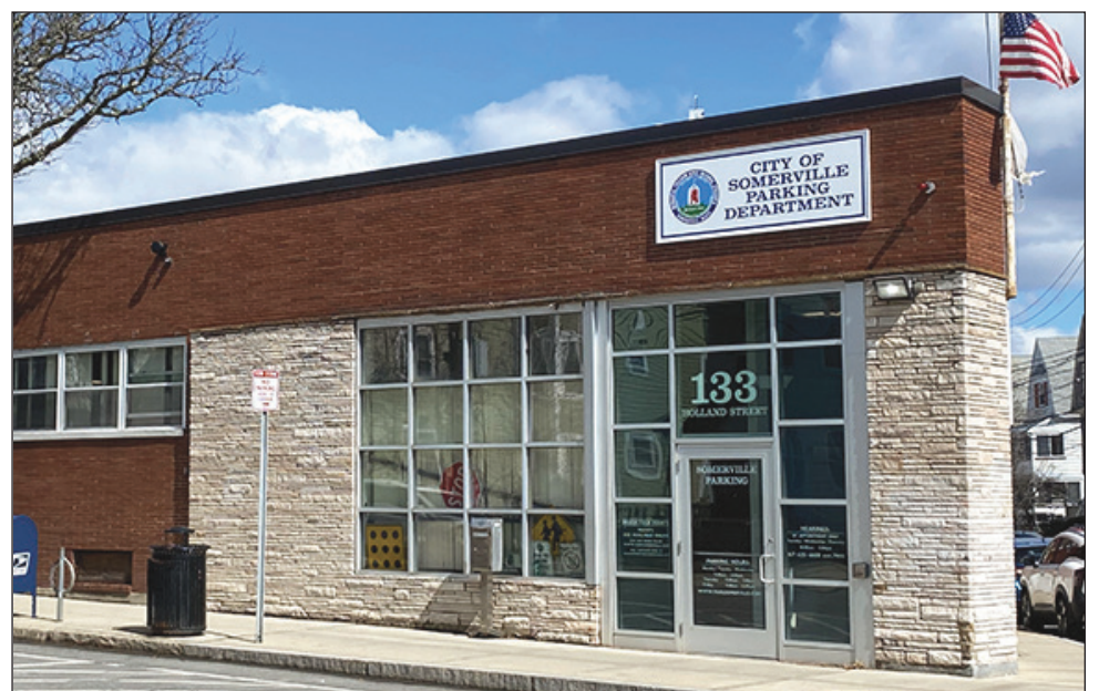
The city’s Parking Office will be the first to go through a decarbonization process to lower costs and help meet climate goals. — Photo by Bobbie Toner
