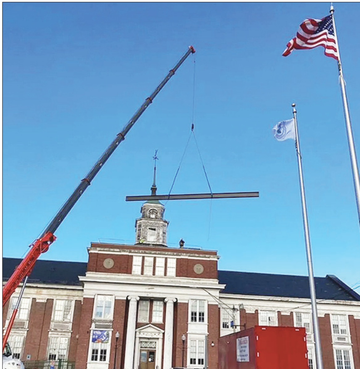
A crane lifts an I-beam to begin repairs to the clock tower at City Hall.
