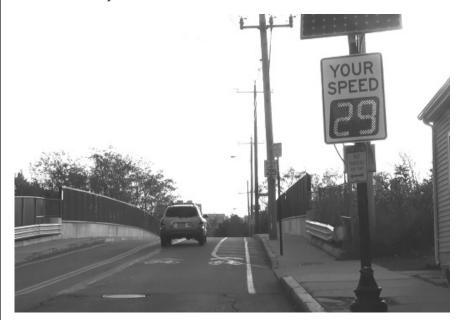
After a serious car crash this May, the city painted a "chicane," a wedge-shaped painting on the asphalt meant to encourage cars to zigzag, thus slowing traffic.
