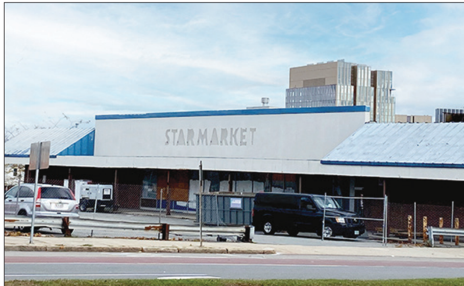
136 affordable housing units are slated to be constructed at 299 Broadway, the site of the former Star Market. — Photo by Bobbie Toner
