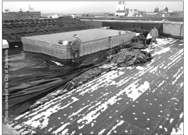
In the wake of Hurricane Sandy, temporary covering was put in place on the Somerville High School rooftop to prevent further damage to the auditorium below.
